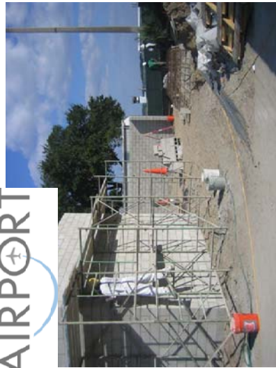
Masonry wall construction – pump house
